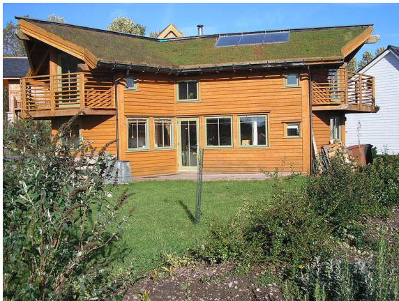
Eco-house at Findhorn Eco village with a turf roof and solar panels
